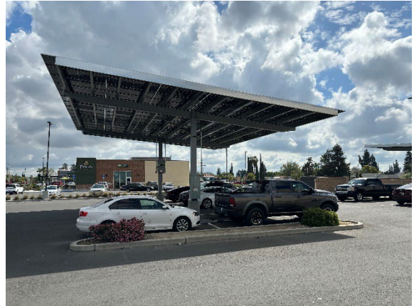
Shared parking lot
